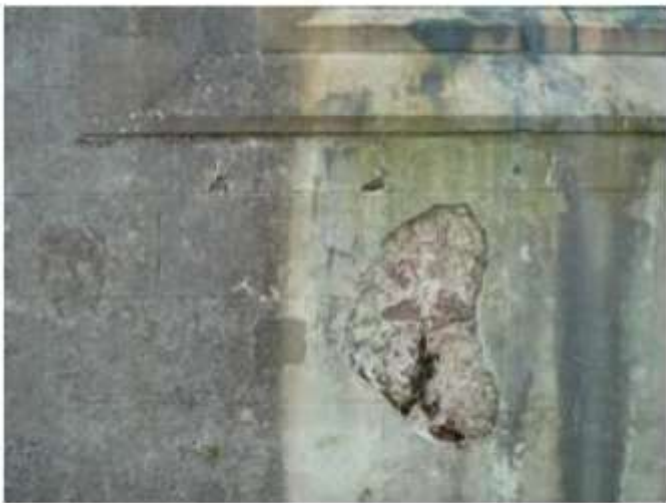
HARLING REMOVED FROM EAST GABLE TO REVEAL STONEMWORK
