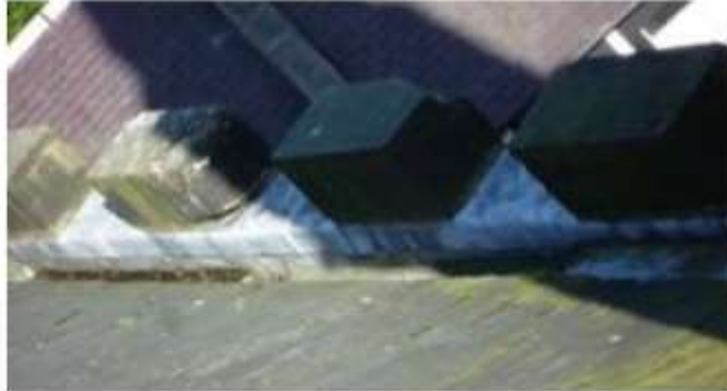
PARAPET GUTTER EAST SIDE OF NORTH TRANSEPT SUNKEN SOLE
