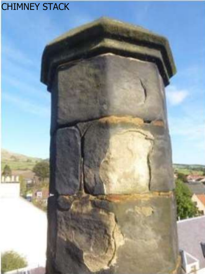
OPENING JOINT THRO MASONRY
