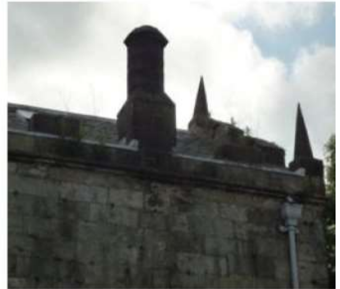
CHIMNEY ON PARAPET OF EAST WALL OF NORTH TRANSEPT
