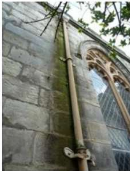
HARLING REMOVED FROM EAST GABLE TO REVEAL STONEMWORK
